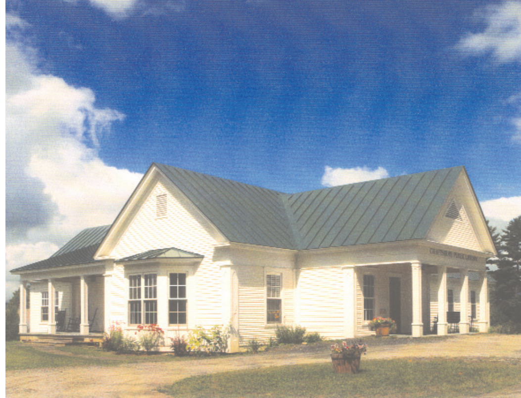
Sited just off the town common, the Craftsbury Library was designed by Sandra Vitzthum drawing from Roman precedents. The entry is a miniature temple front with an oversized porch, designed to welcome all who enter from the common. Significant features include a bay window in the meeting room and a reading porch looking out on the Green Mountains. Photo: Carolyn L. Bates
